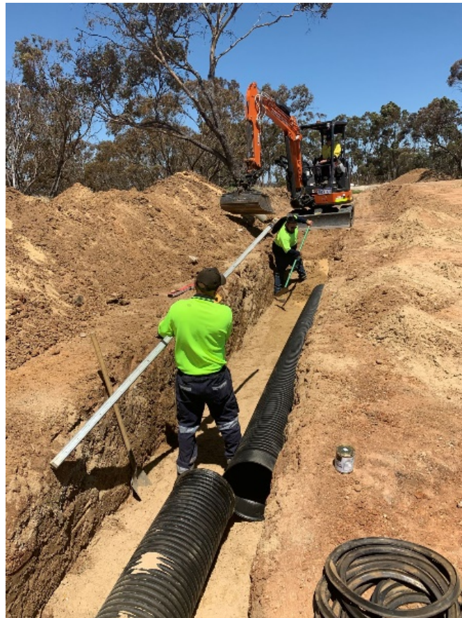
Replacing drain from Gnowangerup Complex oval to dam
