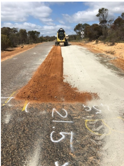
Cement stabilising patches
