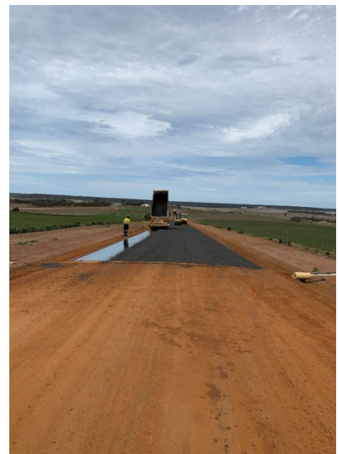
New seal going down on Chillinup
