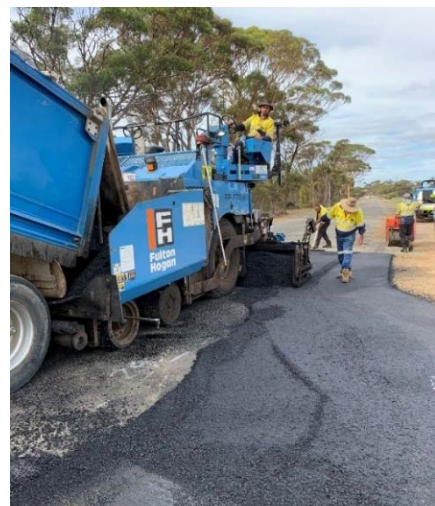
Asphalting intersections on Garnett Road near CBH
