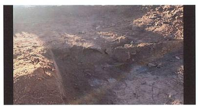
Removal of the existing culvert and replacement recommended with the use of 375 mm SN08 HDPE culverts and precast concrete headwalls.
