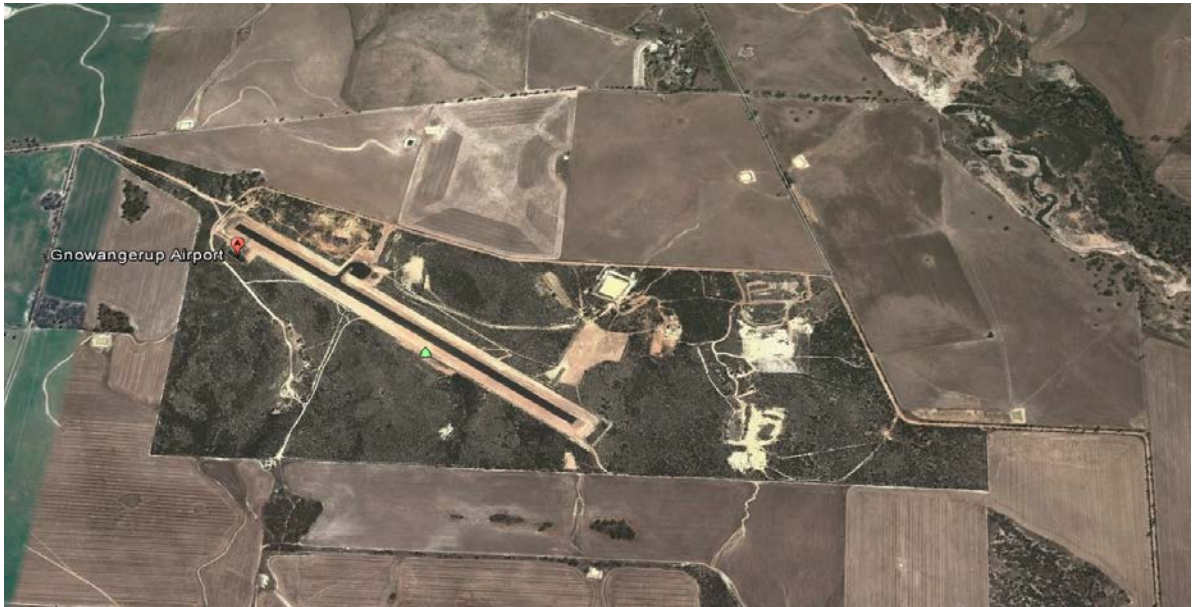
Gnowangerup Airport and surrounds (Image from Google Earth)
