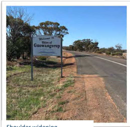
Shoulder widening Gnowangerup - Tambellup Rd
