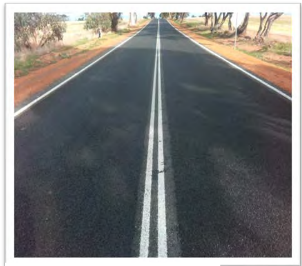
Kwobrup Road finished project
