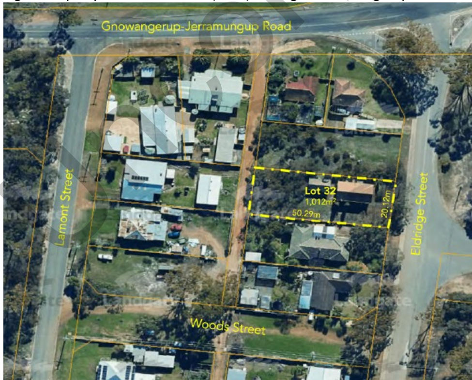
Fig 1 - Property location – Lot 32 (No.6) Eldridge Street, Ongerup
