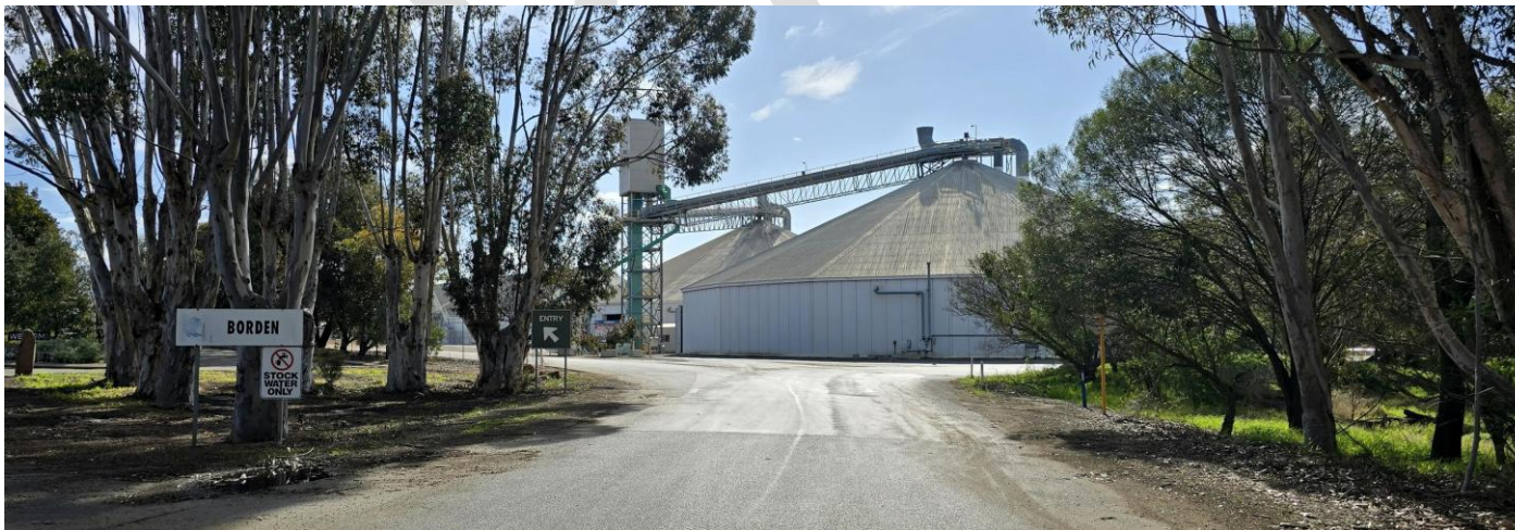
Image: Entrance to CBH facility at Borden
