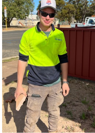
Photo: Shire employee Lewis Claassen who was working hard at doing repairs.
